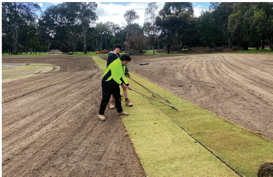
After the existing cool-season fairways were topmaked, six hectares of Santa Ana couchgrass was laid in maxi rolls across 13 fairways over a two-week period before Christmas
