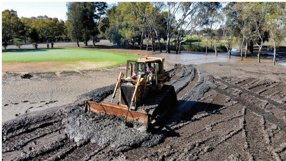
A swamp dozer was brought in after the second major flood to help shift built up silt deposits on the worst fairways
