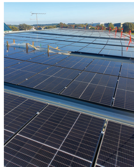
A 100kW solar panel system has been installed on the clubhouse roof at The Sands Torquay, along with a 50kWh battery to capture excess energy
