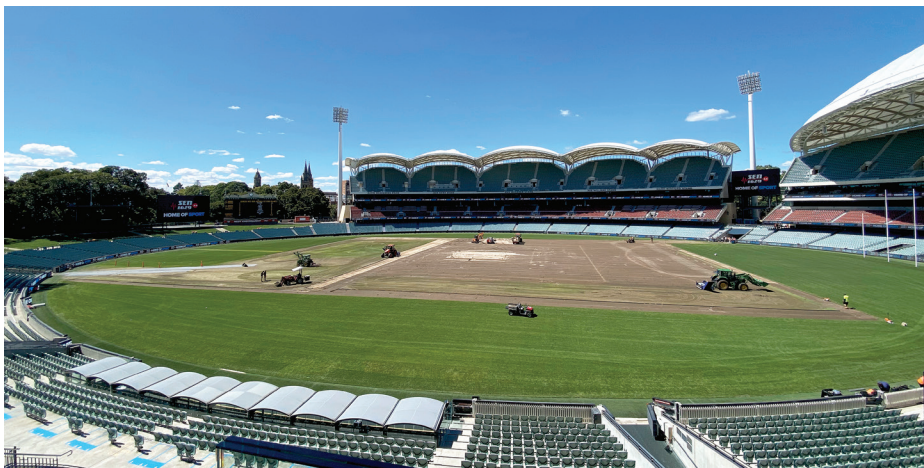
Following the concert bump out, a 10,000m 2 section of the ground where the stage had been was stripped, aerated and re-levelled ahead of turf installation by HG Turf
