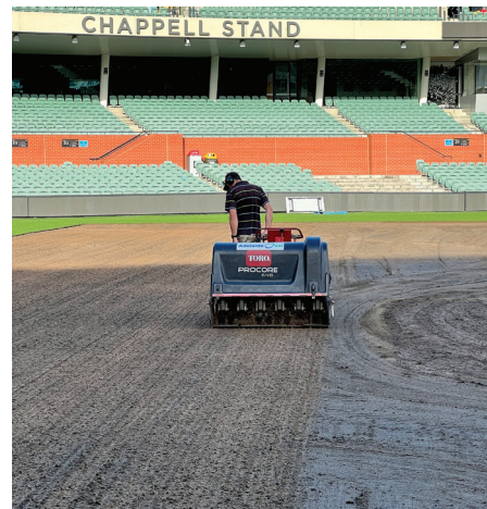
Following the concert bump out, a 10,000m 2 section of the ground where the stage had been was stripped, aerated and re-levelled ahead of turf installation by HG Turf
