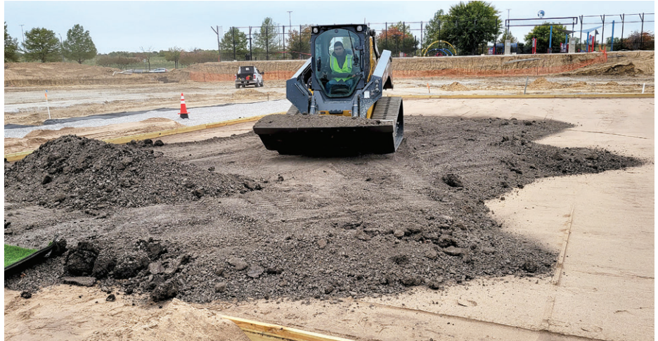
The Grand Prairie Stadium wicket square consists of a 125mm-deep USGA sand layer with a 150mm compacted clay layer. The clay is Pro's Choice ProMound which is used to build pitcher mounds for baseball
