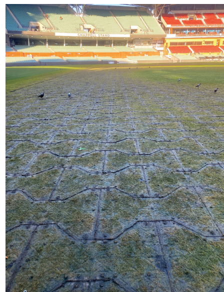
The condition of the centre area of the Adelaide Oval surface after the protective flooring had been lifted
