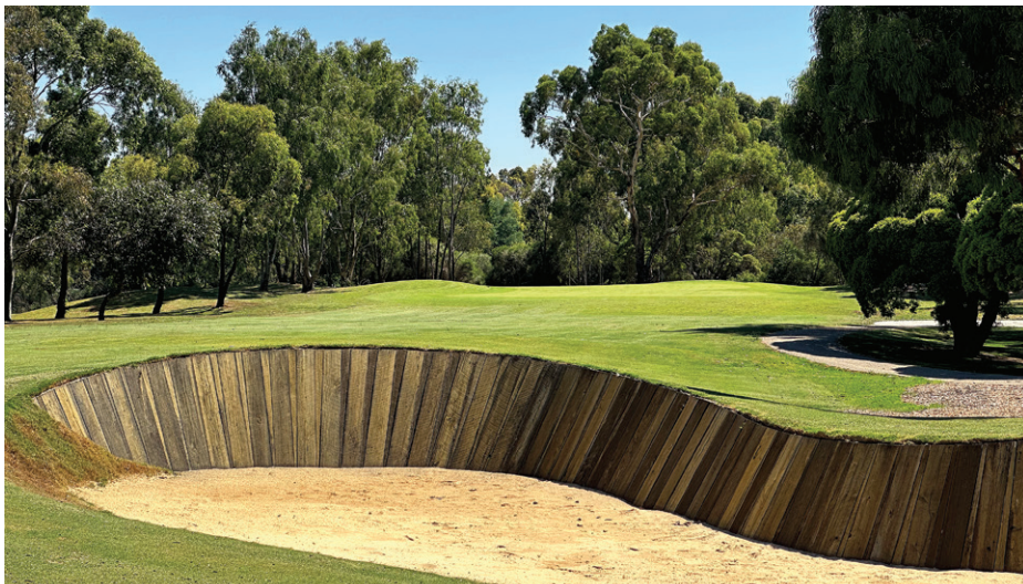
A major component of the Freeway Golf Course redevelopment was reconstructing all bunkers. That included replacing the old sand faces with timber sleepers, creating a unique and striking look throughout the course
