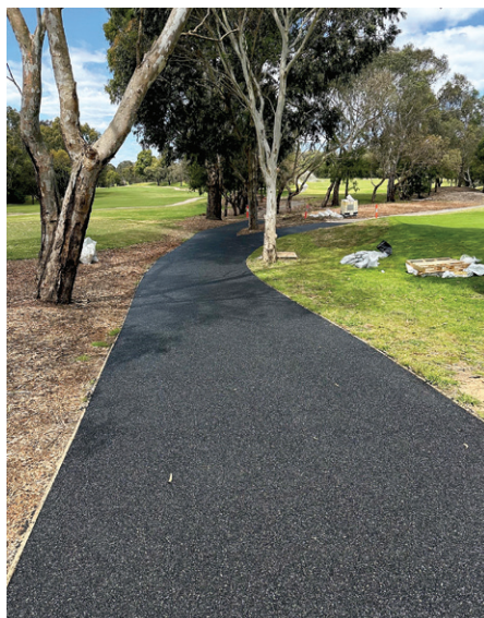
Porous Lane path mix, which comprises around 60 per cent recycled car and truck tyres, being installed at Freeway Golf Course
