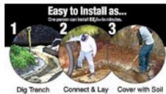
Combining the pipe, aggregate and mesh in one unit reduces the cost of installing a French Drain system by 50% or more. And it eliminates gravel.
