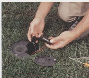
Remove solenoid, wire connections, pilot valve and adjustable regulator...
