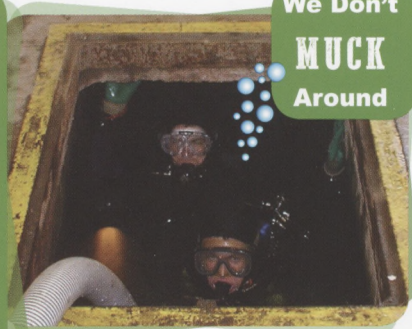
Removing sediment from a wet well
