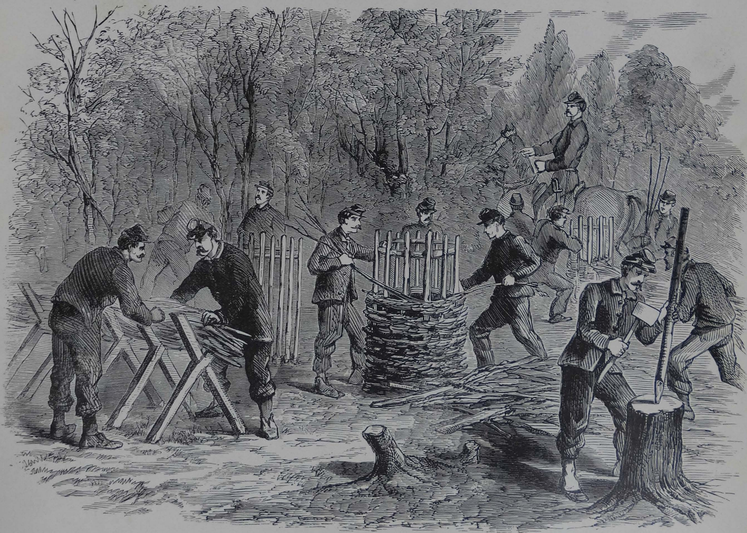
CAPTAIN MULLER'S BATTERY COMPANY OF THE SEVENTY-SEVENTH PENNSYLVANIA REGIMENT MAKING FASCINES AND GABIONS FOR BREASTWORKS.
