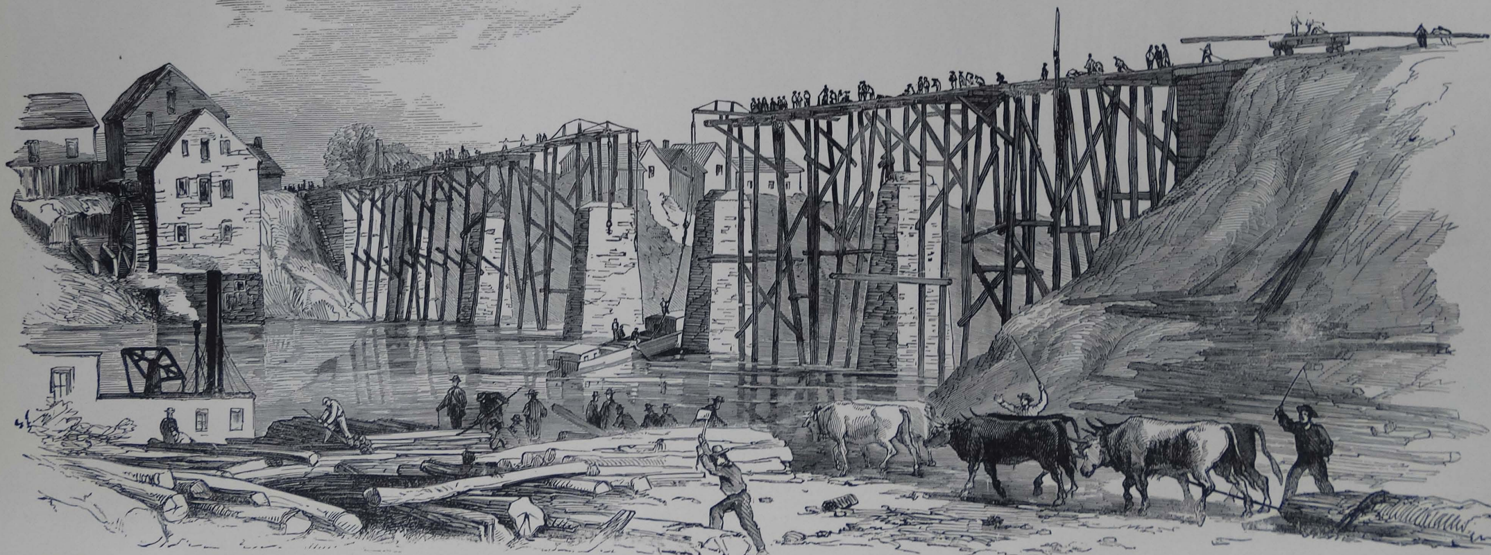
REBUILDING OF THE RAILROAD BRIDGE OVER THE RAPPAHANNOCK TO FREDERICKSBURG, BURNT BY THE CONFEDERATES IN THEIR RETREAT FROM FALMOUTH, APRIL 19th, 1862. FROM A SKETCH BY OUR SPECIAL ARTIST, EDWIN FORBES.
