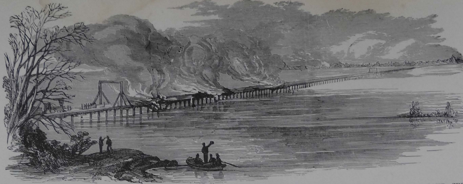
BURNING OF THE GUNPOWDER CREEK RAILROAD BRIDGE, ON THE PHILADELPHIA AND BALTIMORE RAILROAD, BY THE MARYLAND SECESSIONISTS.
