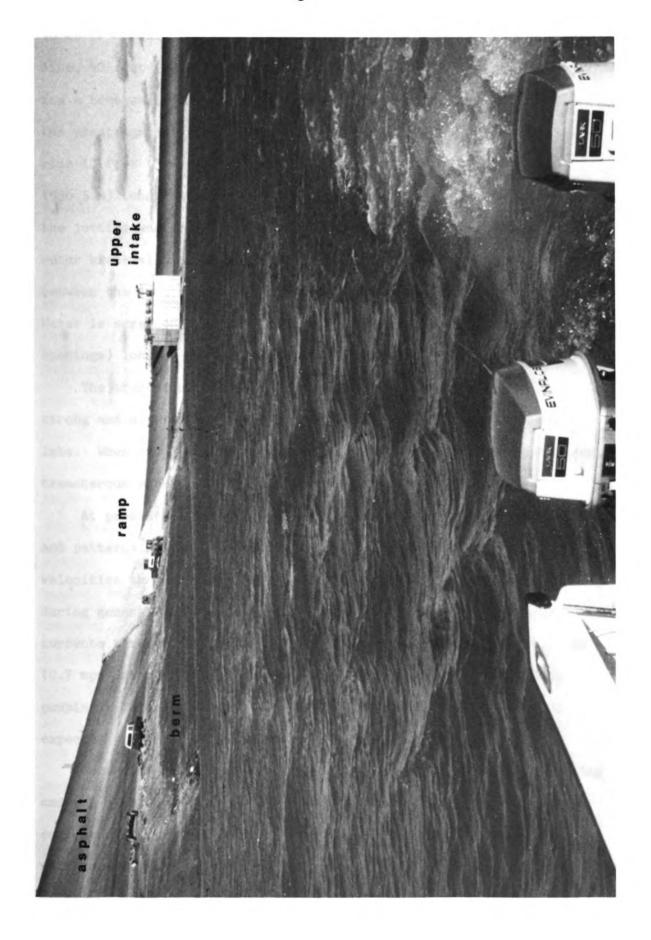
30 meter depth. The lower intake structure is adjacent to the shoreline, 40 feet (12.2 m) below the water surface. Two large jetties
