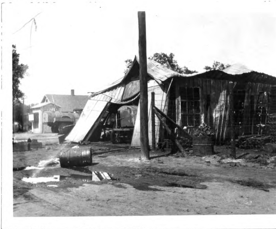
This photograph illustrates the effects of an explosion of gasoline vapor in a bulk oil station pump house in Wichita, Kansas. The vapors were ignited by the arc from an ordinary enclosed knife switch used to control an open single phase motor.
