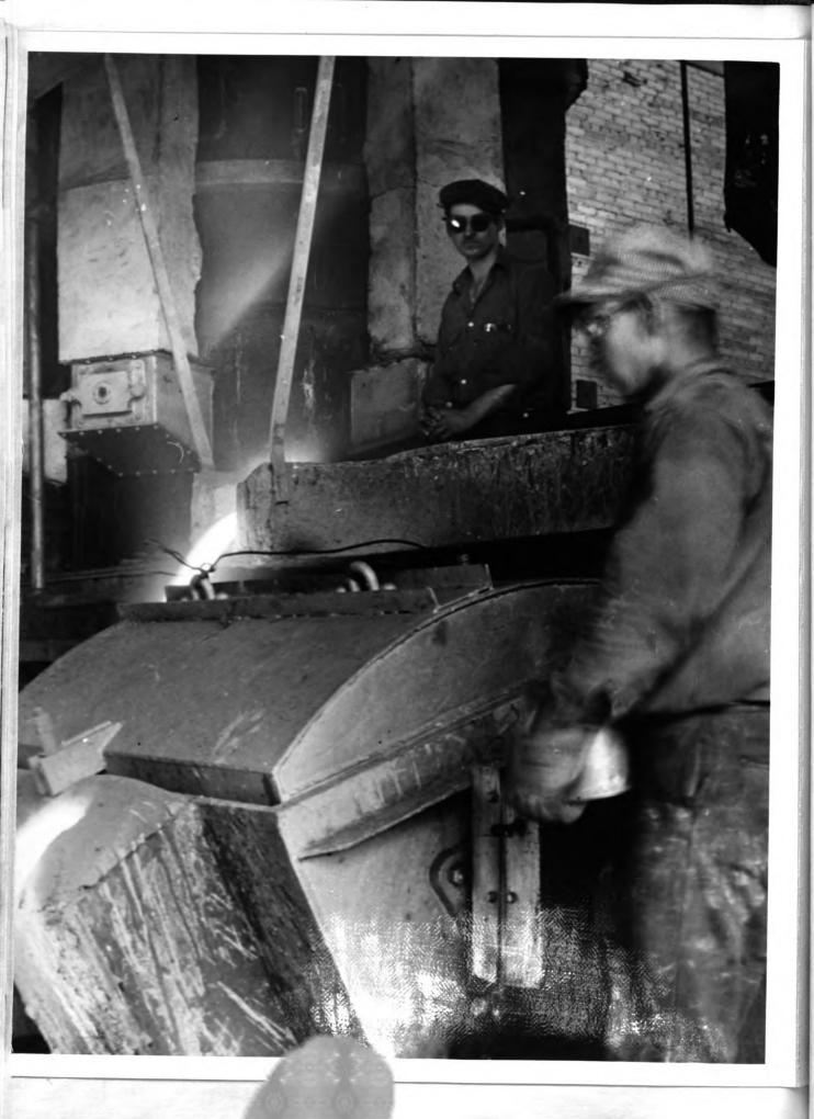
Tapping iron from cupola into mixing and de-sulphurizing ladle, then into delivery ladle.
