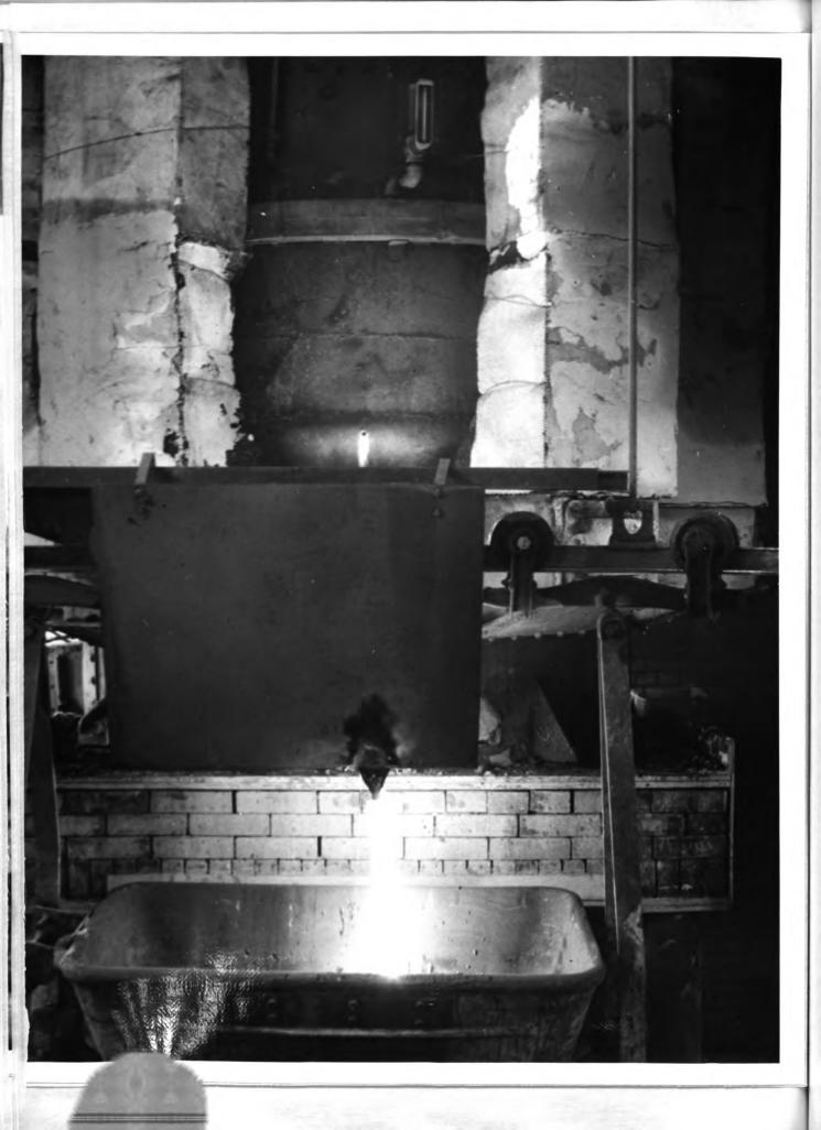
Cupola (72 in. dia. shell, lined to 54 in. dia.) rear view showing slag running into slag pot.
