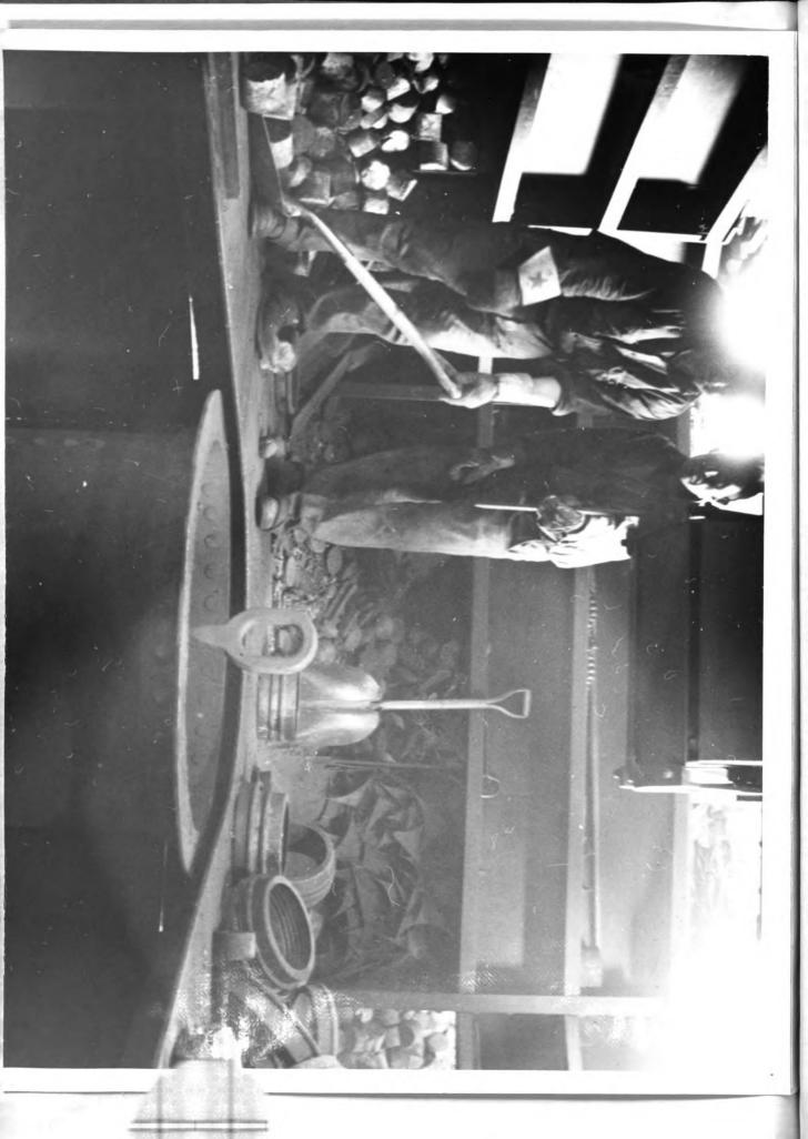
Charging bins and coke hopper, showing cone type charging bucket in place on scale, ready to be filled.
