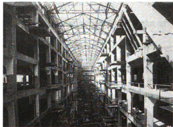
Figure 4.6 Construction photo of the interior of the extension factory with reinforced concrete columns.
