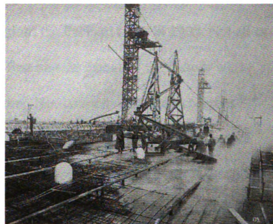
Figure 4.4 Construction photo of workers pouring cement over a wire frame, creating a strong, reinforced concrete floor.
