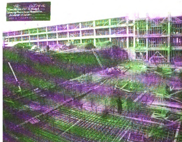
Figure 4.11 Photo showing the construction of the foundation of the new power house in 1916. In the background is the construction of the new AA extension building.
