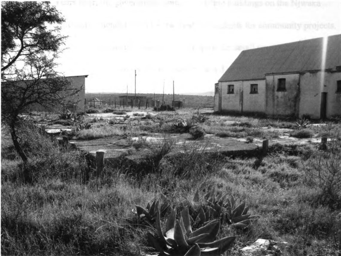
Figure 10: The factory foundation in the church yard as it appeared in 2008 (photo by the author).
