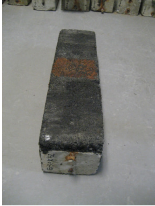
Figure 2.17: Specimen with Waterproofing and HMA Overlay
