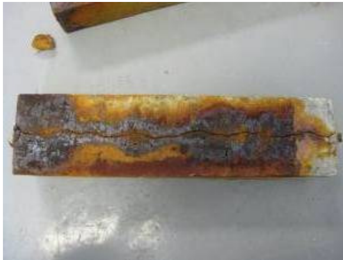
Figure 2.13: Specimen after Level 4 Corrosion
