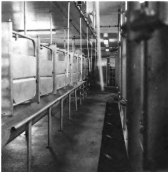
Figure 2.22B System "ON"- All Feedgates Closed Except #1
