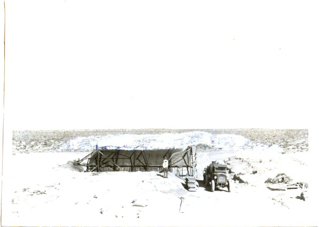
Curing of Magazine Arch.
