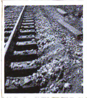
Figure 3 Skeletonized Track by Power Cribber
