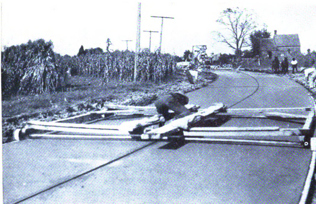
View showing joint finisher edging the slab.
