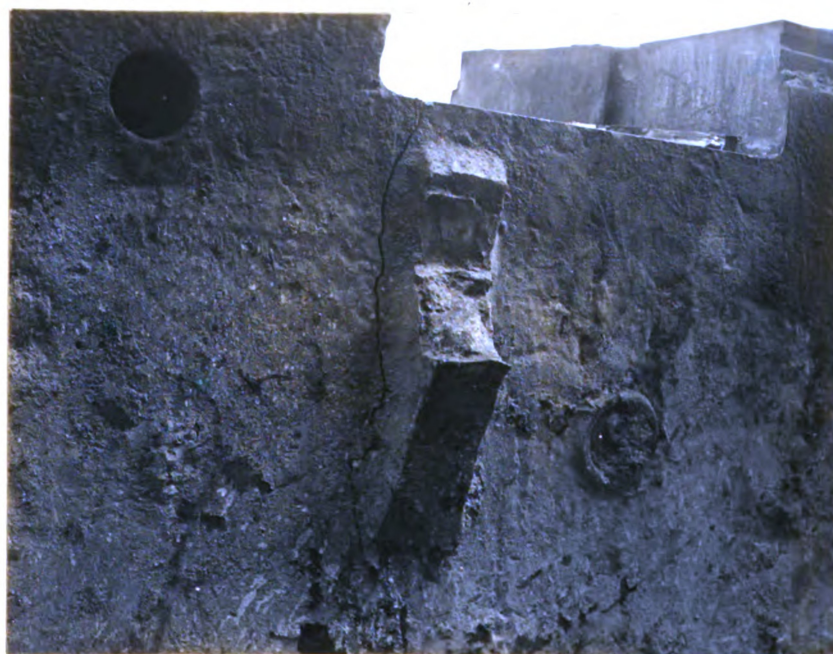
Figure 1. Typical hammer base failures.
