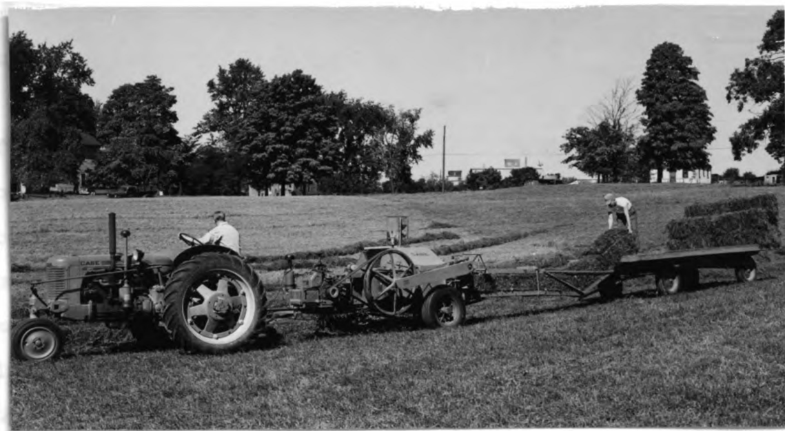
Fig. 3. Automatic twine tie baler in action
