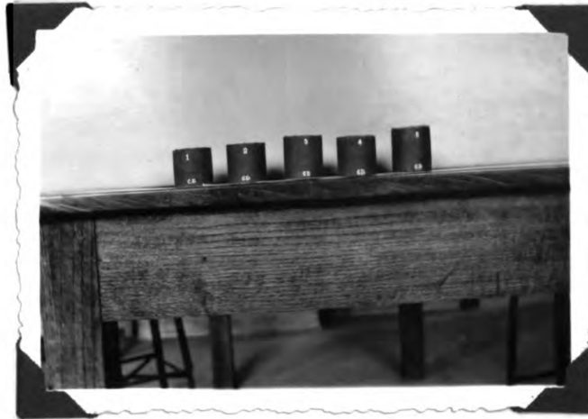
Fig. 8. Coarse Sand & Clay with Varying Asphalt Content--lab. dried.
