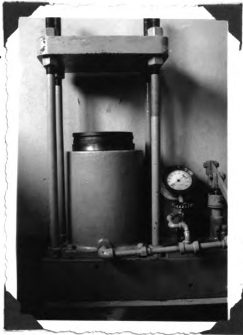
Fig. 1. Compression Machine.
