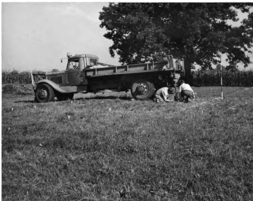
Method of conducting bearing test.
