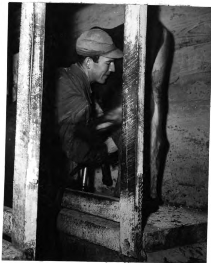
Figure 16 The operator puts a milking unit on a cow that has been previously prepared. One operator handles two long tube milking machines in this four stall elevated milking room.
