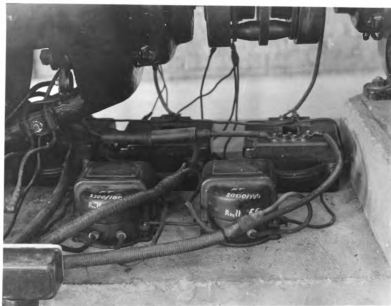
Instrument Transformer Connections
