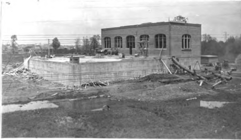
New pumping station and reservoir under construction.
