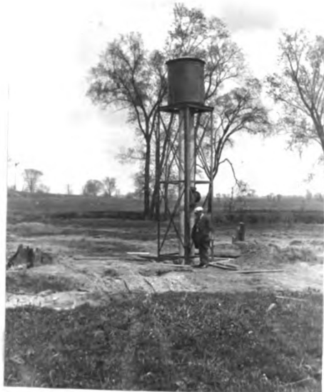
Air lift well ready for operation.
