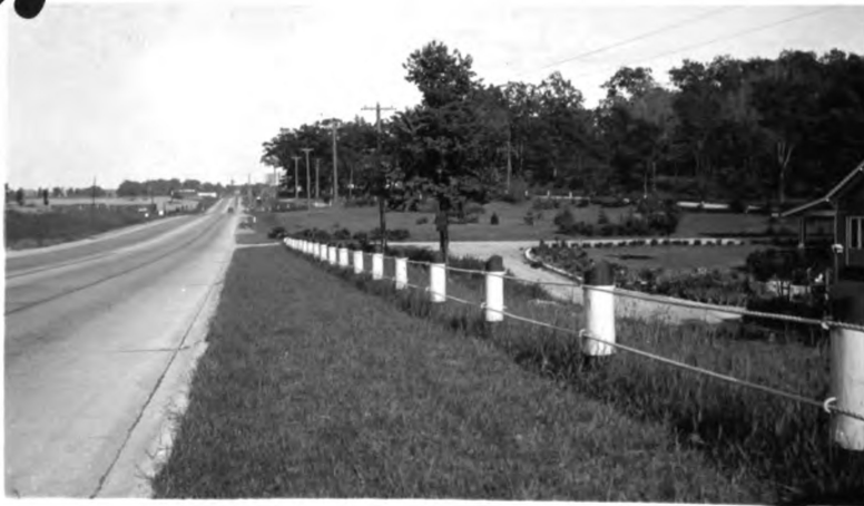
Okemos Corner looking east from Grade separation 6.9.32 P.V.
