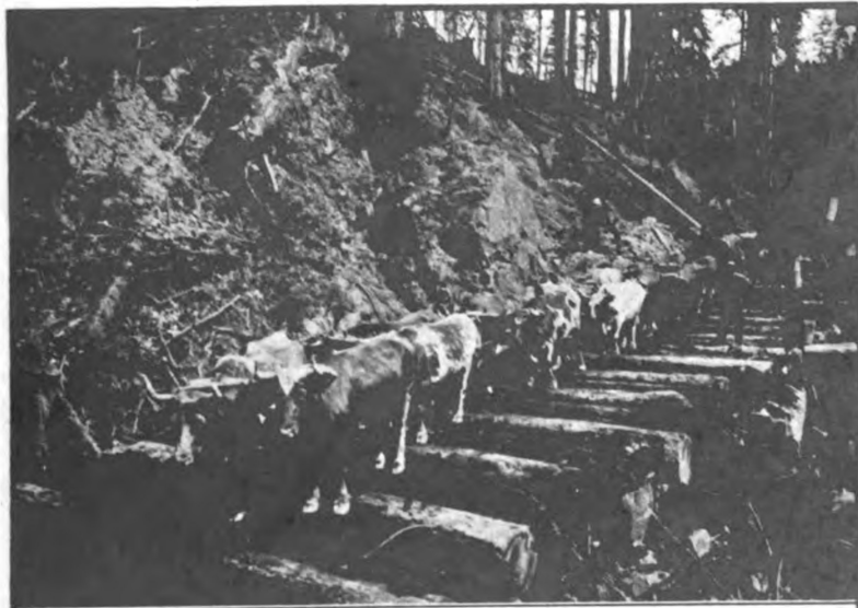
Corduroy roads were among the first "all weather" roads in the United States. The one shown here was used for redwood logging operations in northern California.
