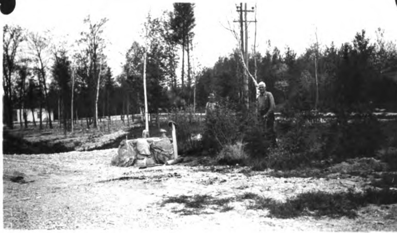
Landscaping spring North of Oden, looking South. Maint. Sec. 31-2, Emmet County. J.W.A. 5-24-32.
