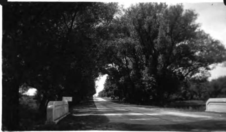
M-60 Willows and bridge over Sandstone Creek 7-1-32 G.E.M.
