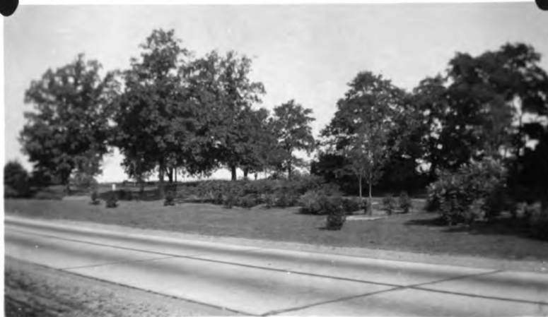
Roadside Park U.S. 112 Hillsdale Co. E. of Jonesville 7-14-32 G.E.M.
