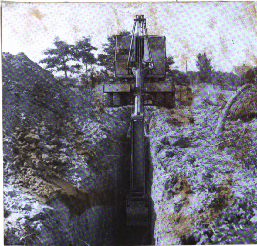
Trench hoe on sewer construction
