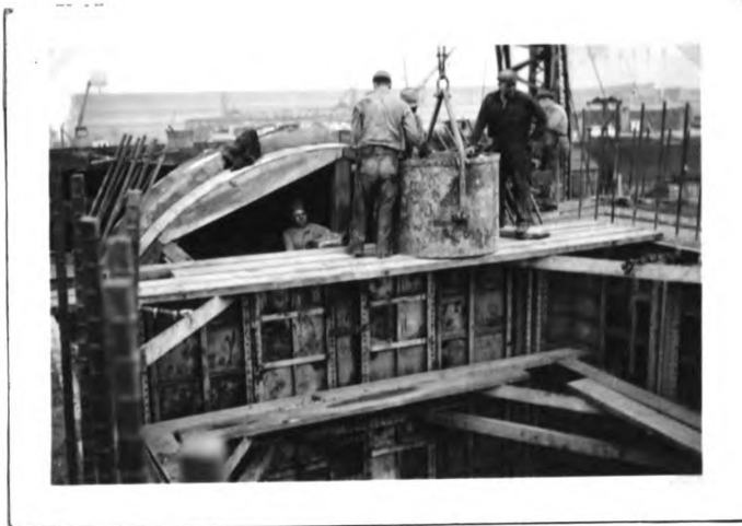
Loading pig-iron in tunnel opening in shaft to balance the weight of opposite side.
