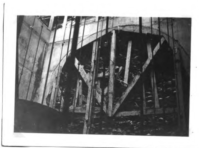
Beginning of the operation of unloading pig-iron from tunnel opening after the shaft has been shouldered to hard pan.
