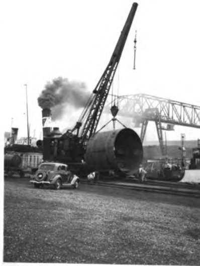
Shield being lifted from barge that it was brought to the site of the job.in.
