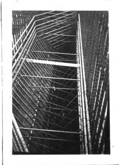
Reinforcing placed in cutting edge. Note complicated and heavy design due to large forces exerted by the great head of earth at bottom of the shaft.
