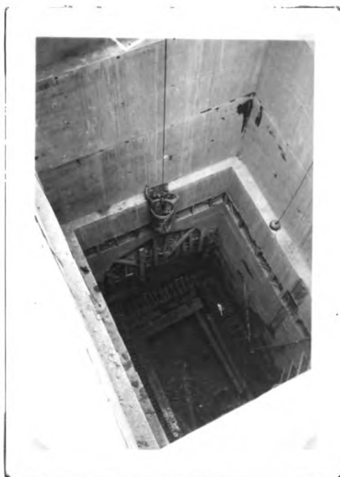
Looking down into shaft after it has completed its decension. Reinforcing for lower deck bent out from shaft wall.
