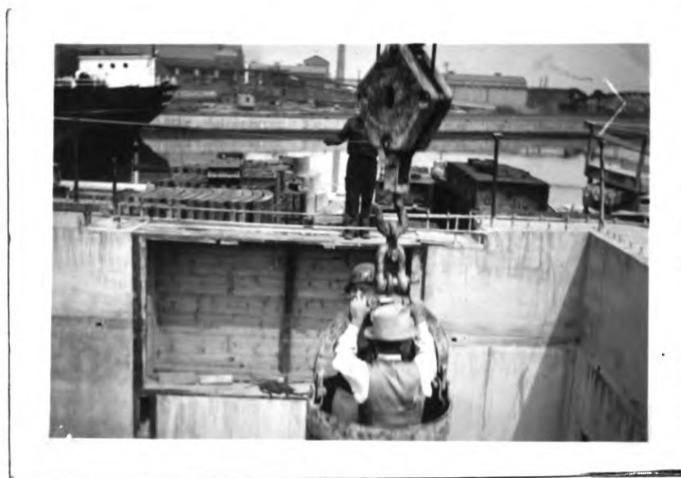
Lowering of workman and inspector down into shaft. Signalman in background.
