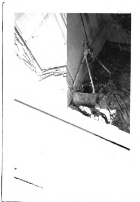
Mucking at bottom of shaft.
