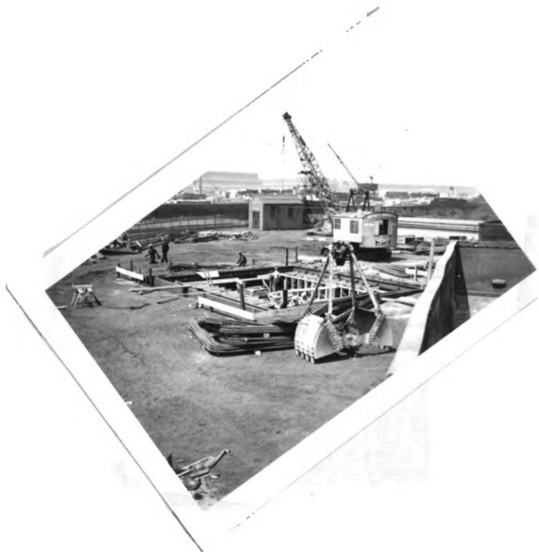
Cutting edge in place - erecting of the wooden forms taking place by carpenters.
