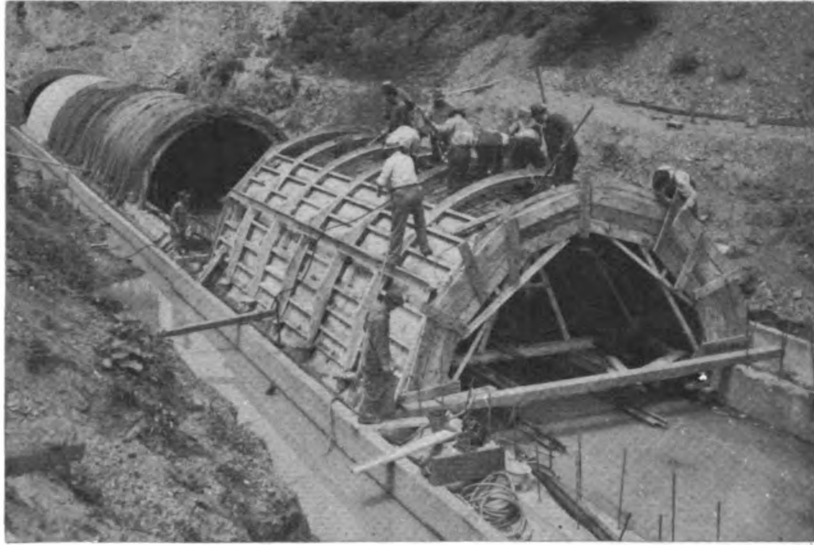
A View Showing Outside Forms on a Sewer.
