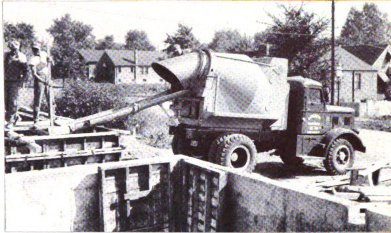
Pouring Foundations with Transit Mixer.
