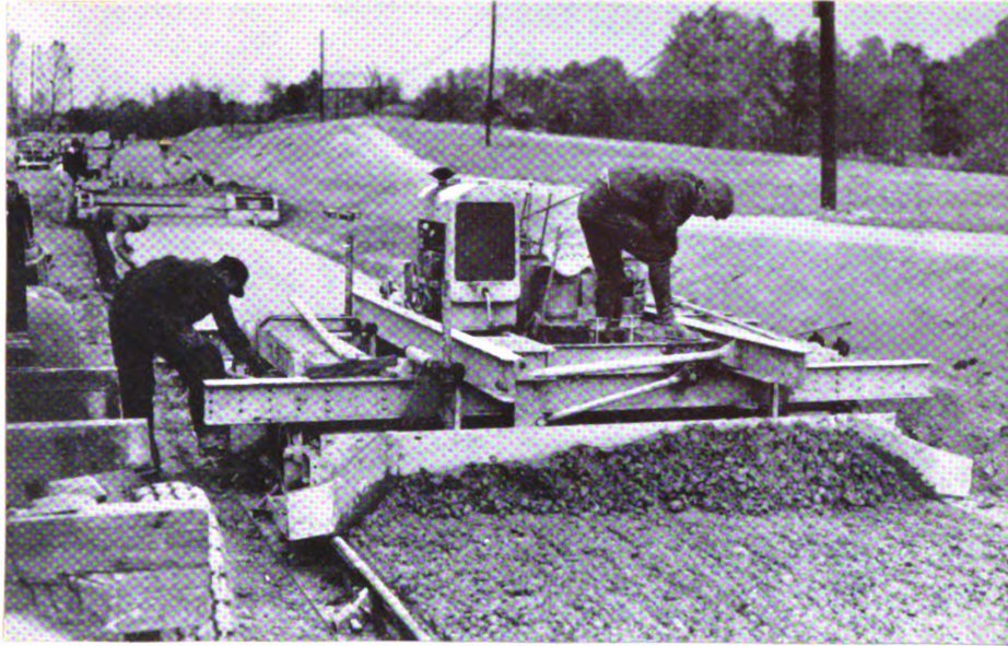
First Pass of a Finisher on 11 ft. Pavement.
