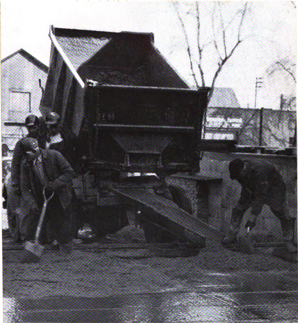
Modified Dump Truck Discharging Concrete.
