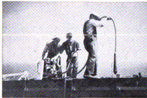
A Vibrator Being Used.
