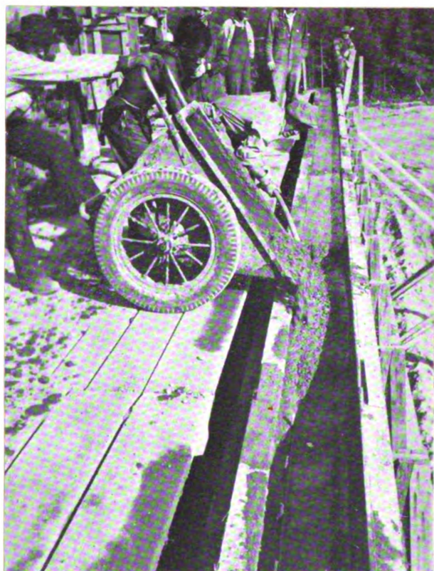
Pouring Concrete with a Buggy.
