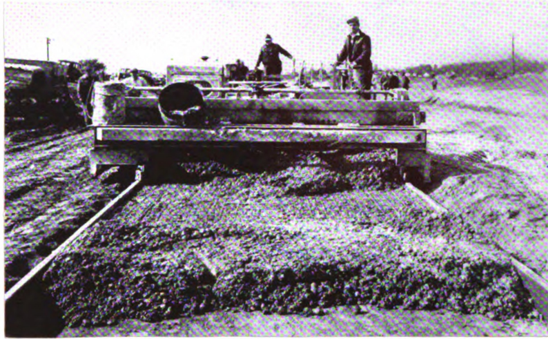
Front View of Spreader on 11 ft. Pavement.
