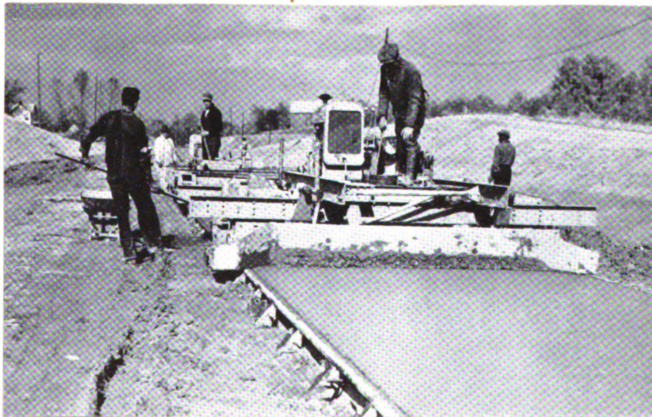
Second Pass of Finisher over the Same Surface.
