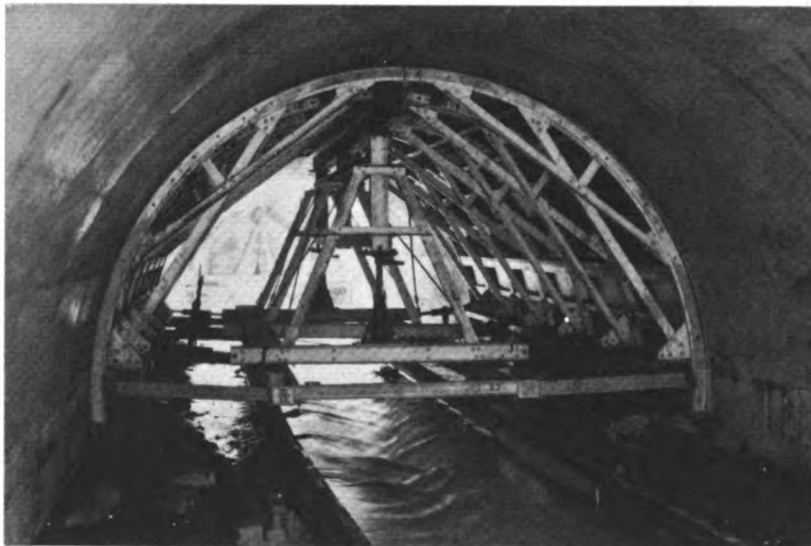
A View of Inside Forms on the Same Sewer.
