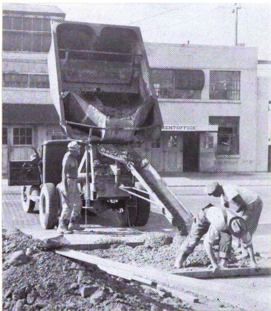
"Dumpercrete" Truck Pouring Concrete.
