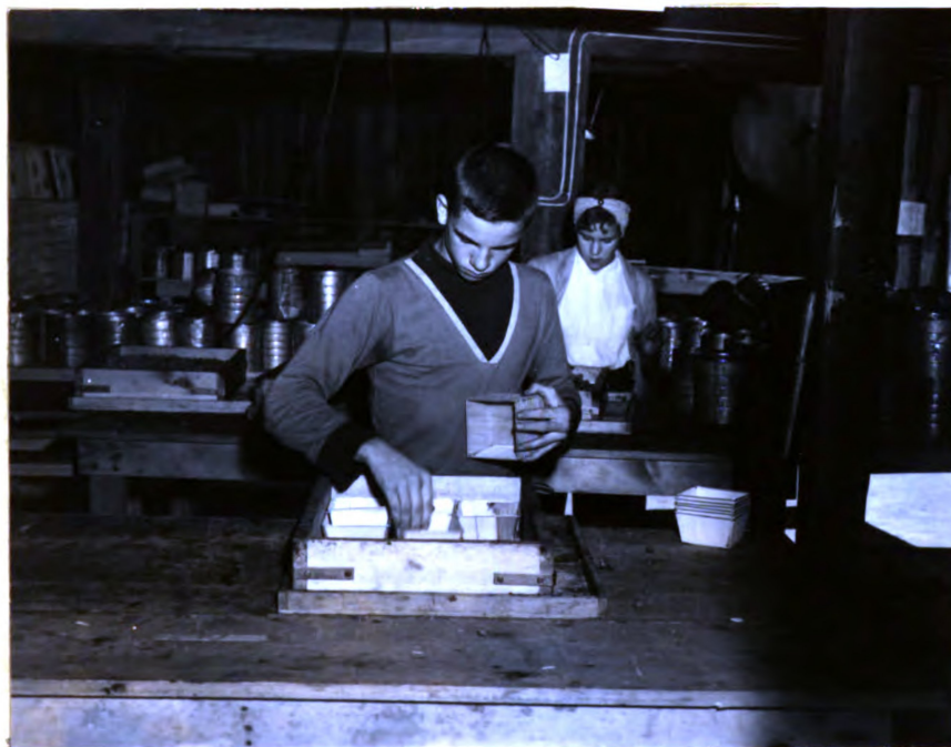
Fig. 20 One worker places frames on trays and places 12 pint cups inside each frame. This work is done on the auxiliary table next to the line.
