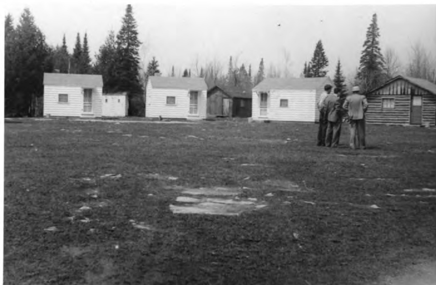
Figure 25. Class 3 site about 10 miles east of Shingleton on M-28. Rock actually appears on surface (foreground) averages only 2-5 inches below. . . . 2.8
