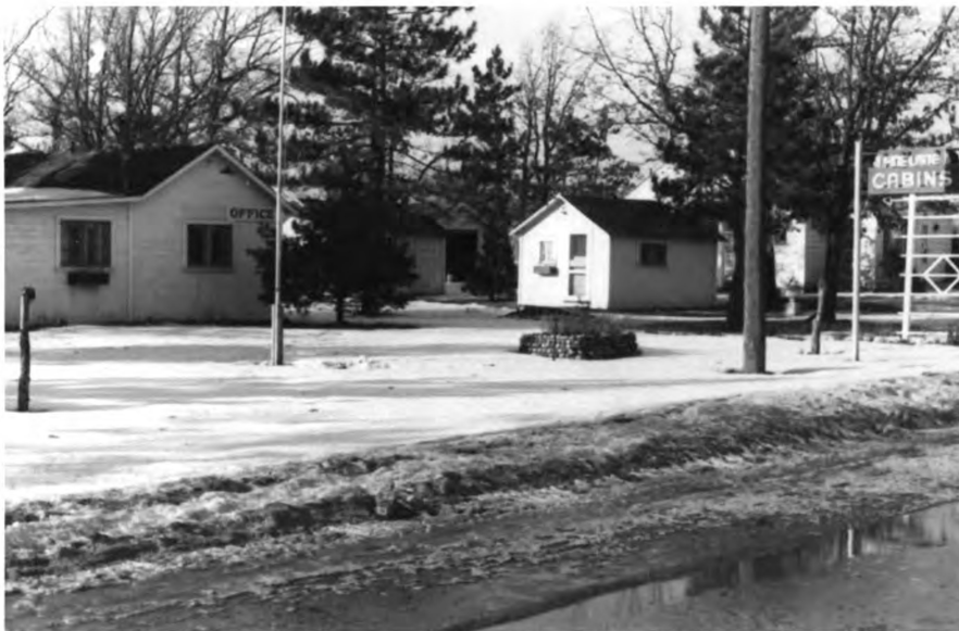
Figure 40. Office and cabins, Pine Lane.
