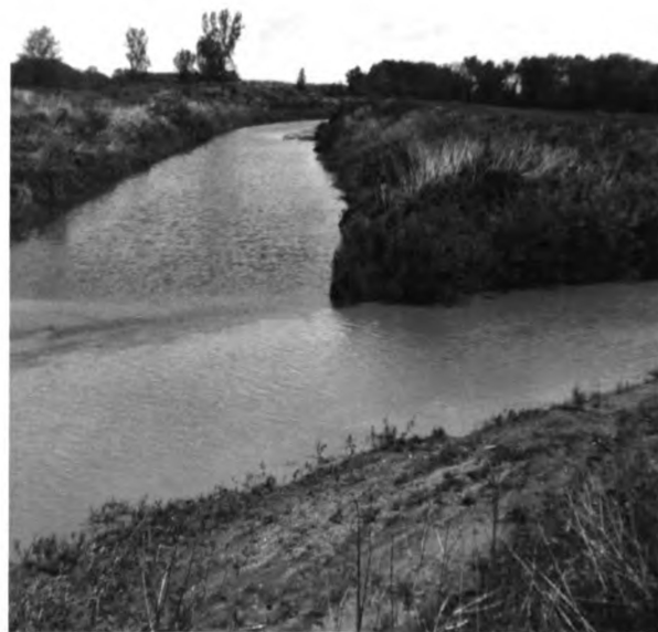
Fig. 9 Looking up the Little River from where it is joined by Little Lile Creek. Both streams have been dredged here and the material spread out so there are no high spoil banks.
