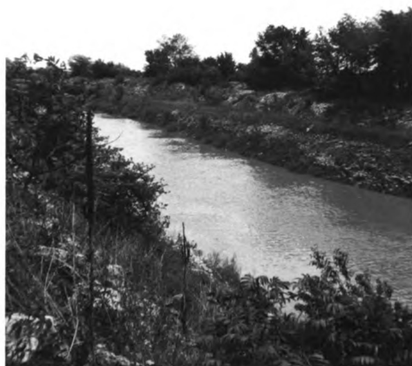
Fig. 8 Little River near Howers town, Huntington County. Note the chunks of limestone that make up the spoil banks here. This portion of the river was blasted through the bedrock.
