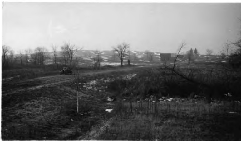
07-19 Hillsdale N. Sta 136-143 OLS 11-30-31 Looking E. Marl deposit in foreground. Sandy gravelly hills in background
