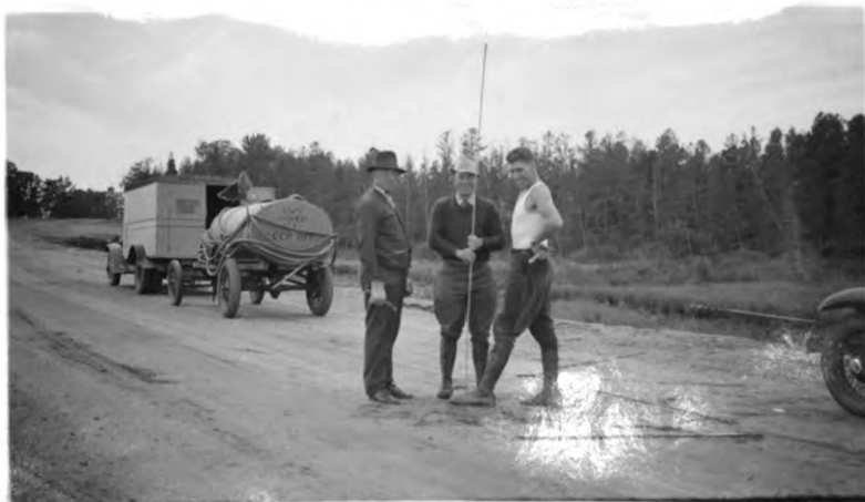
59-7 Cl Schoolcraft Reloc. Sta 60 Stokstad Dry boring thru fill to sample marl. Tarley's outfit. 9-22-32
