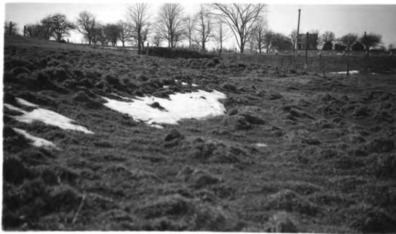
059-27 Sheridan So. 2-23-33 Stokstad Sta 327 R. Boggy condition of side hill indicates seepage.
