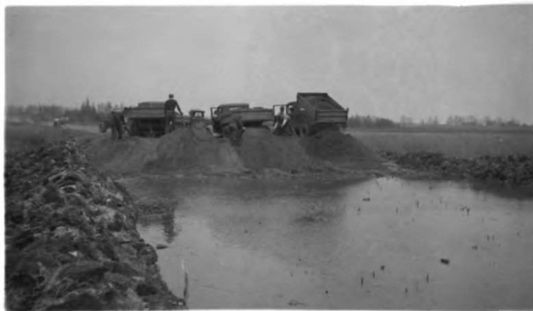
03-701 Schoolcraft Reloc. Sta 63 3' sand fill on 33' marl. No heaving ahead or at side of fill. 3-20-32 Rudolph
