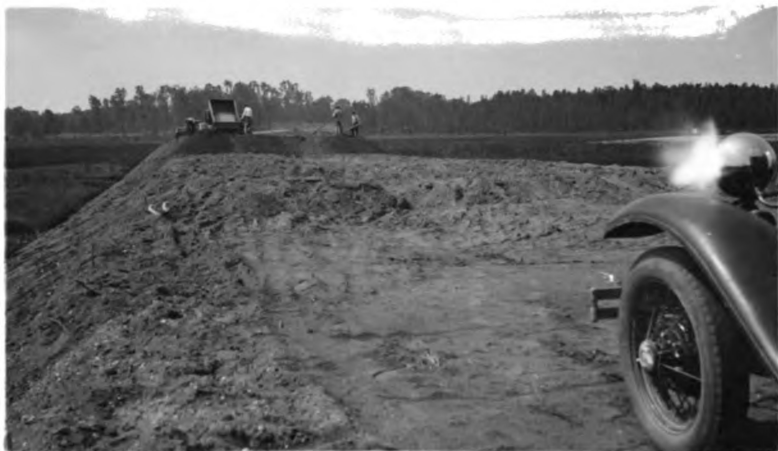
7-7 01 Schoolcraft Reloc. 3-10-32 Stokstad Sta 69. Placing surcharge accelerated settle- ment here. 4th lift across in 2 days.
