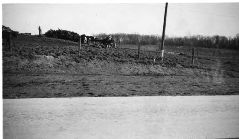
059-27 Sheridan So. Stokstad 2-23-33 Boggy Condition on side hill indicates seepage - Sta 336 R.
