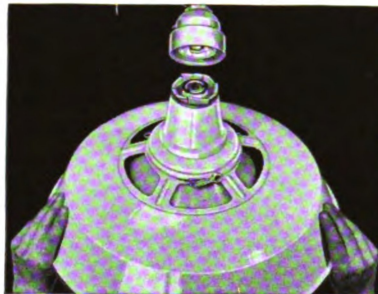
A single trip up the ladder—the quick, easy exchange of a previously cleaned reflector for the dirty one
