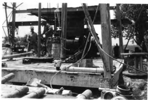
Rotary equipment drilling for gas in tri-township field.
