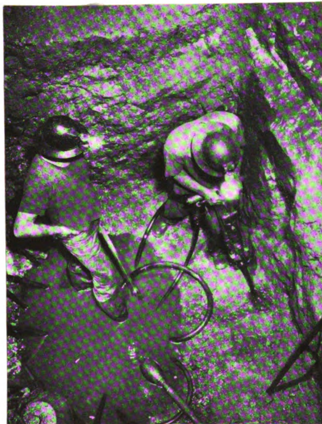
Sinker Drill Operating in Shaft Illus.1b
