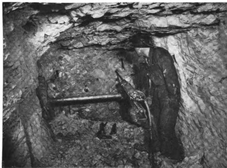
Drifter Mounted on Horizontal Crossbar Illus. 2b
