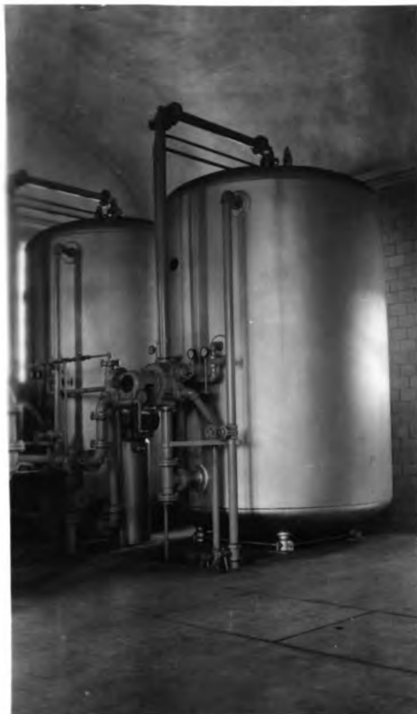
Iron Removal Tanks.
