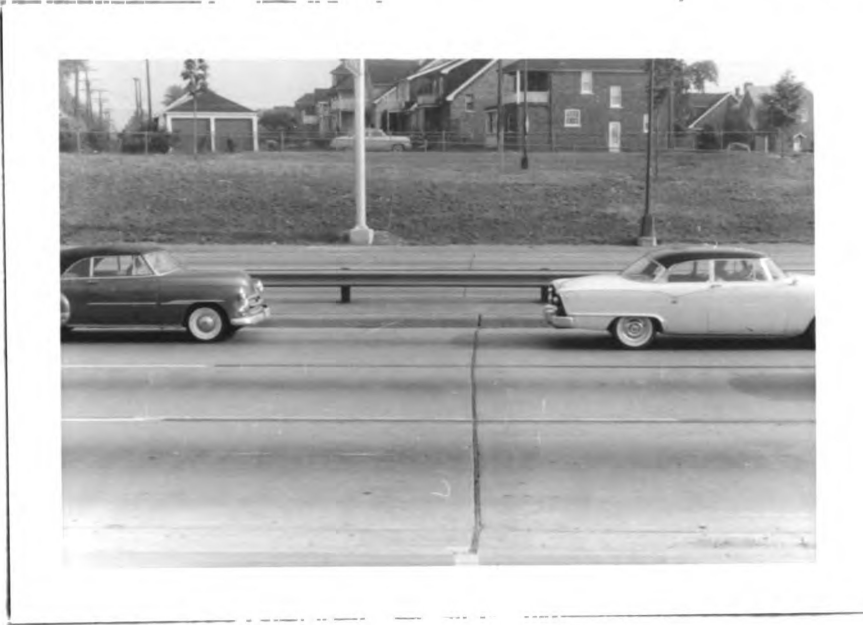
Headway: Edsel Ford Expressway, Detroit. Note the minimum headway between these cars, actually less than twenty feet, at speeds between 50 and 60 MPH. Time spacing of these cars is approximately 0.3 seconds.
