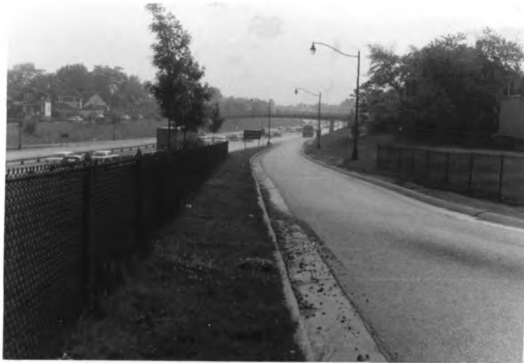
Ramp, Edsel Ford Expressway, Detroit. View shows the Ramp is void of any frictional features and is long enough to provide for attaining speed of expressway and proper merging when headway is ample.
