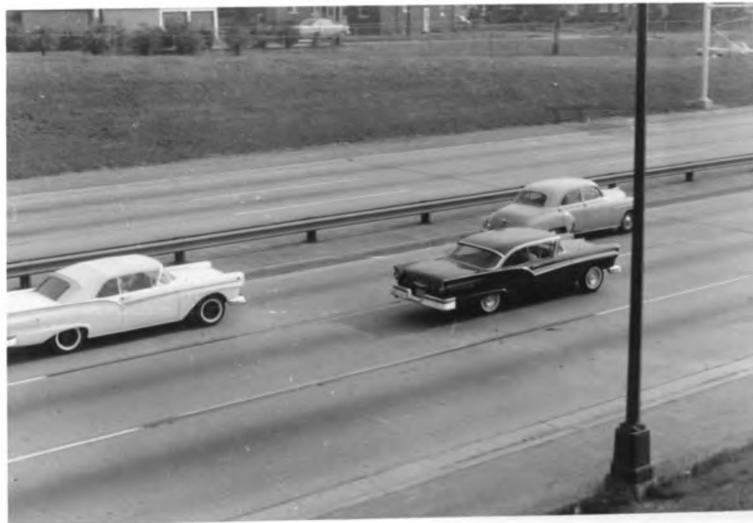
Headway: Edsel Ford Expressway, Detroit. Note the minimum headway between these cars, actually less than 25 feet at speeds between 50 and 60 MPH in both lanes. Car in the center lane has little effect on spacing.
