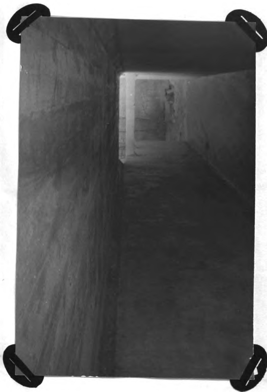
Flume looking downstream
