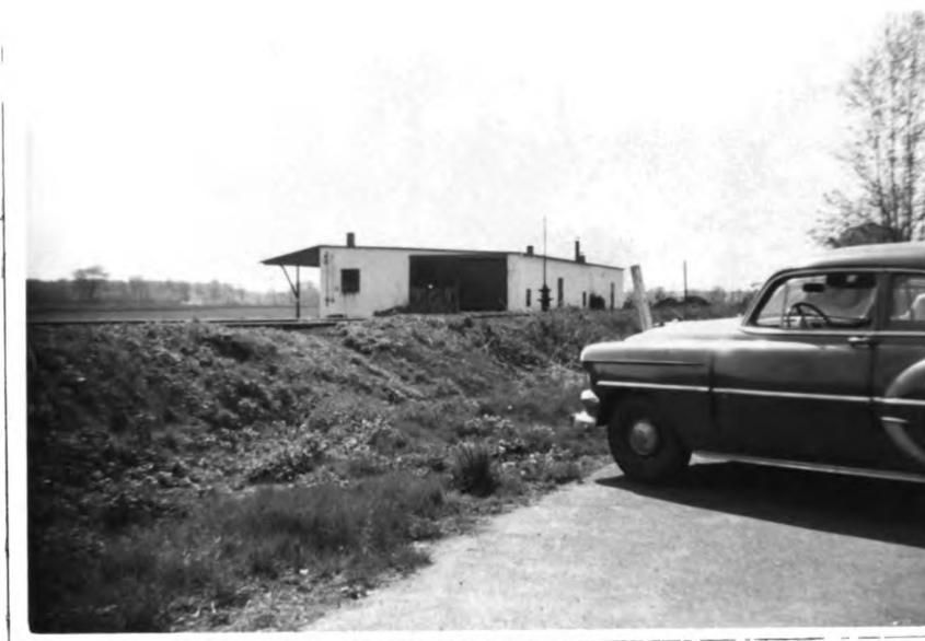
Figure 60. Co-op warehouse in Hooper. In the foreground are the tracks of the spur of the N. Y. Central Railroad.
