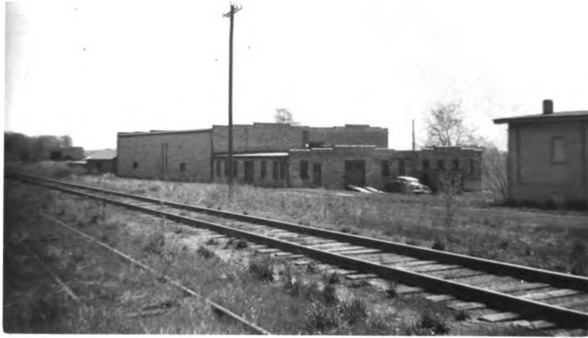
Figure 53. Cold storage warehouse in Martin. Operated by a food product company for storage of fruit purchased from fruit growers near Lake Michigan.
