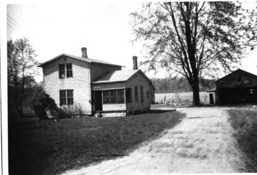
Figure 64. Another migrant labor housing facility.
