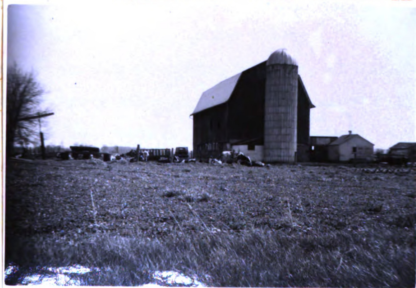
Figure 24. The dairy barn of the Fenner Farm. Note the resemblance to the Jackson barn. It is similar to almost all the dairy barns in the area.
