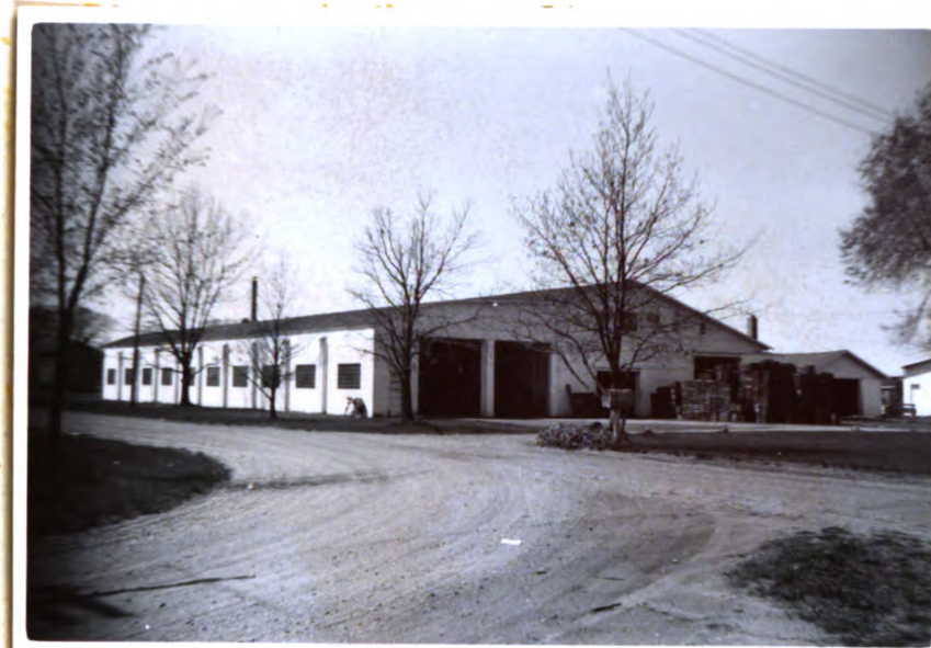
Figure 32. Potato storage and grading warehouse. It is located near Orangeville.
