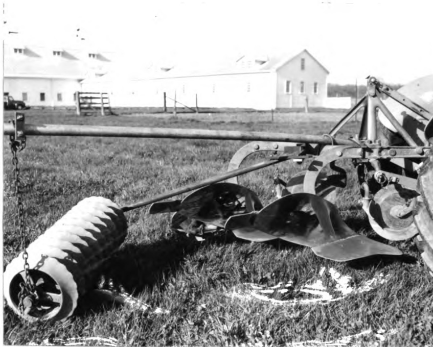
Fig. 9. The cultipacker unit about to be lifted. The boom is for side support.
