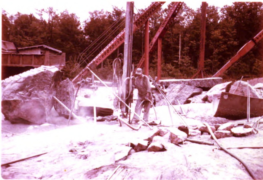
Figure 22 Drill operator at work at the Loon Lake quarry.
