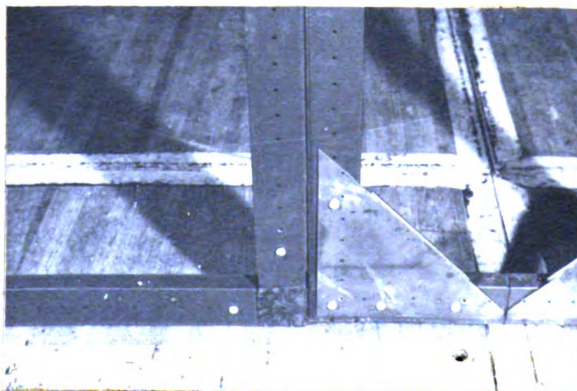
Figure 16. Detail of two methods of making right-angle joints.
