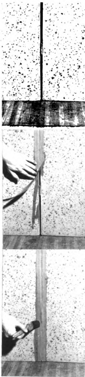
Figure 18. Applying gauze dutchman over L-hinge.
