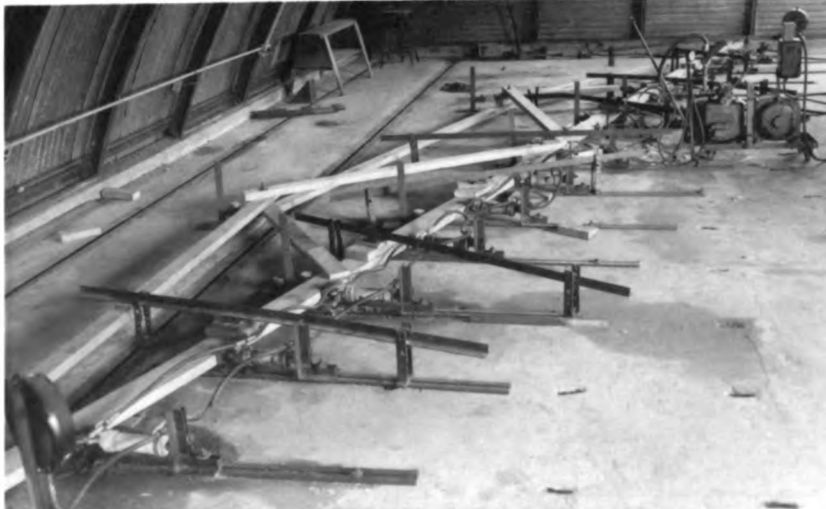
15c - Truss type "B" in place and ready for testing
