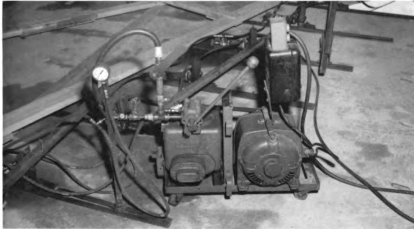
15a - Hydraulic pump and control apparatus used to apply pressure to the trusses
