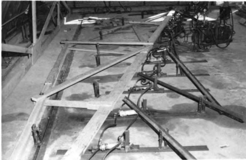
15b - Truss type "A" in place before cylinders and hold-down bracket have been applied
