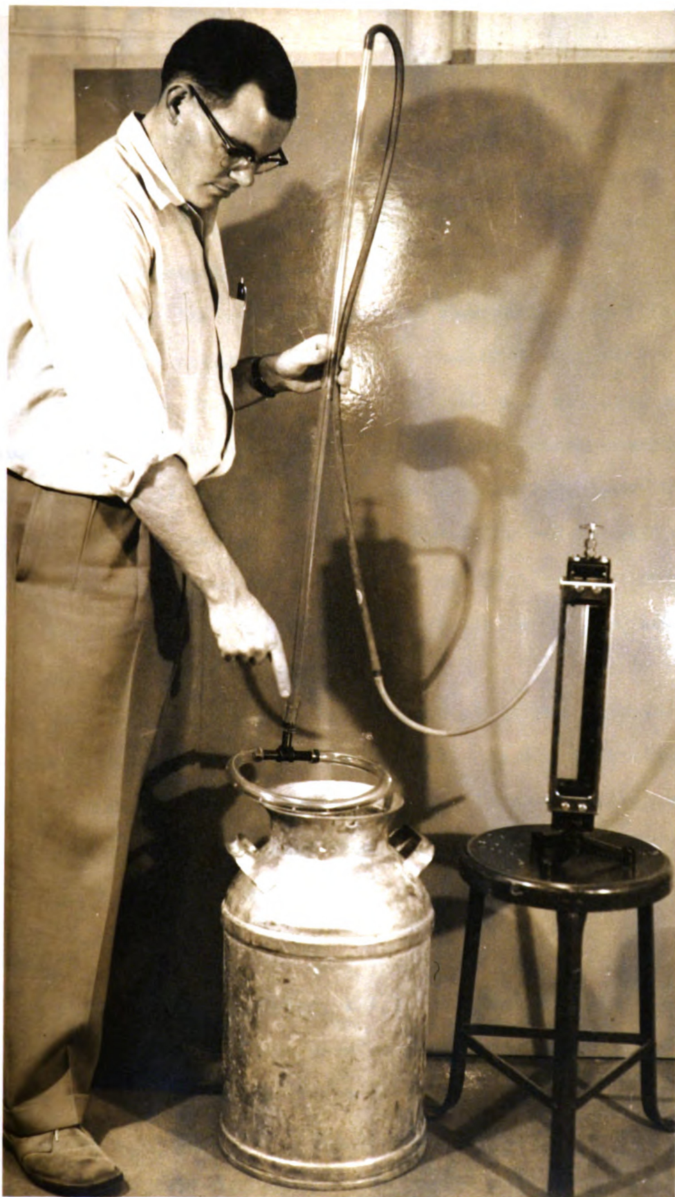
Figure 3. Equipment for agitating 5-gallon samples of milk.
