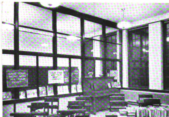
"Sight-saving" classroom; semi-indirect lighting units spaced about 11 feet apart; 300 watt lamps
