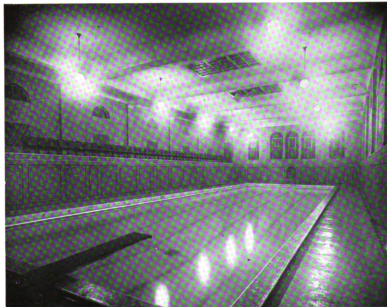
FIG. 16 Night View of a Swimming Pool Lighted by 150-watt MAZDA C Lamps in Round Glass Globe Reflectors. The average intensity is two foot-candles. Note that the lighting equipment is accessible from the edge of the pool, a desirable practice. When properly arranged, lighting fixtures are not necessary over the middle of the pool as evidenced here
