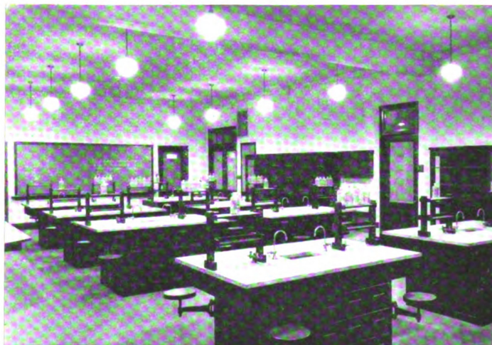
Laboratory; direct lighting units spaced about 10 feet apart; 200 watt lamp.
