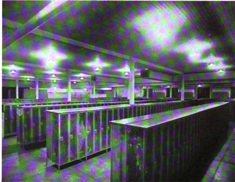
FIG. 15 Night Photograph of a Gymnasium Locker Room Lighted by 60-watt Clear MAZDA B Lamps in Flat Prismatic Glass Reflectors. The room is finished in dull gray paint, and lamps are spaced 8 by 14 ft. located close to the 11-ft. ceiling
