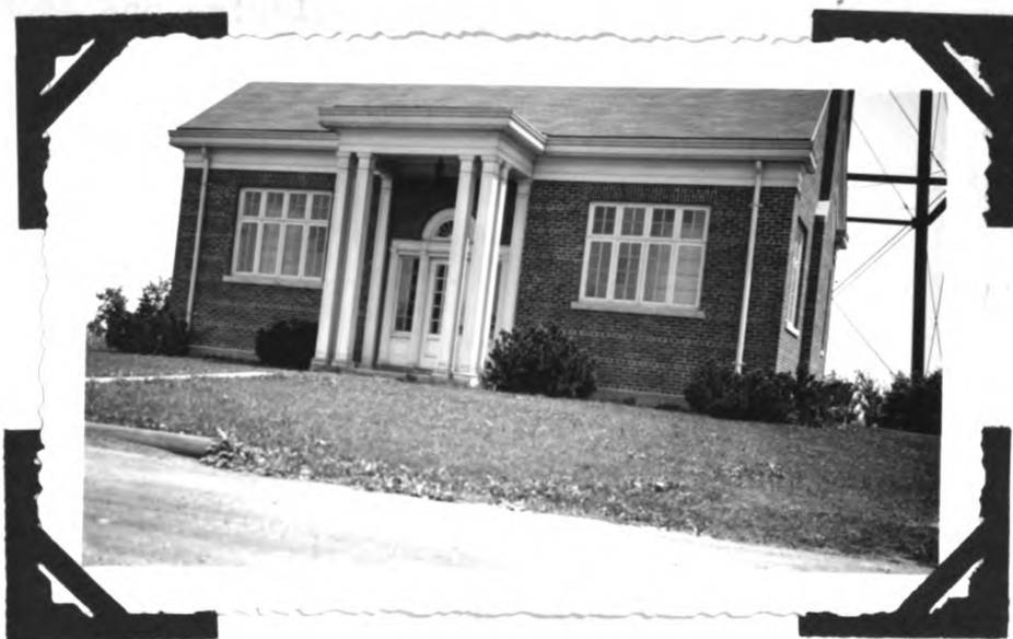
East Lansing Water Treatment Plant
