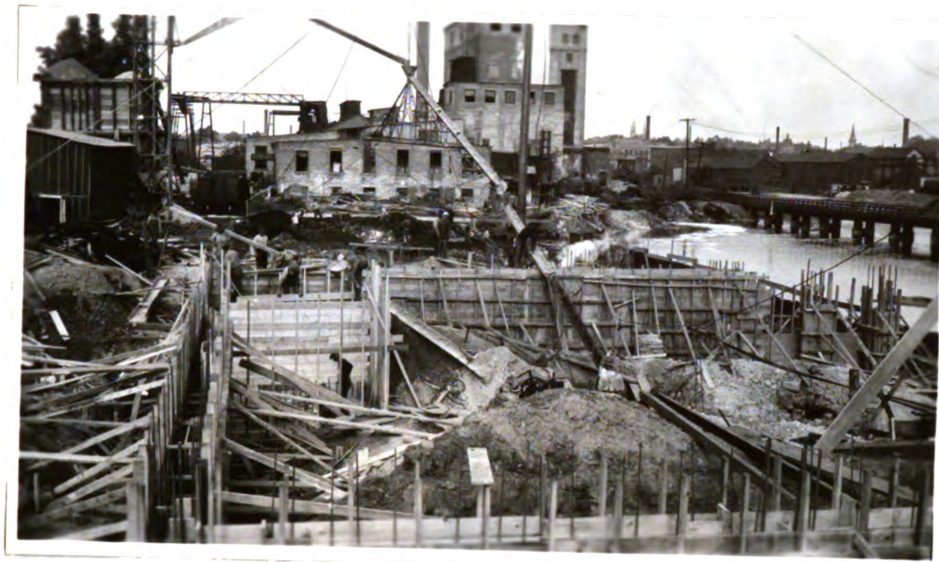
#9 August 17, 1923. Forming for water wheel pit, Excavating for machine bldg. piers.
