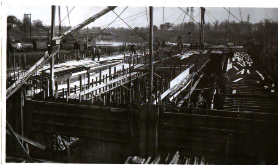
#21 Oct. 23, 1923. Forming main or paper machine floor of machine building. Machine pit partially formed at left.
