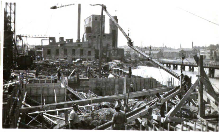
#10 August 17, 1923. Showing method of pouring the south wall of finishing building.
