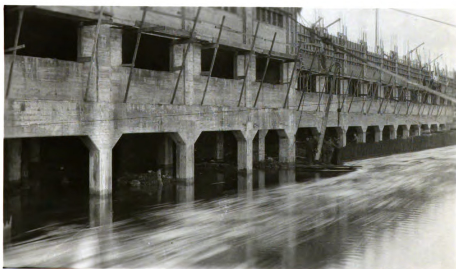
#22 Nov. 9, 1923. Pulling sheet piling. Block and tackle, breast derrick mounted on raft.
