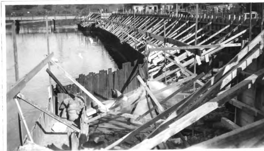
#15 Sept. 14, 1923. Cribbing and cofferdam. Method of bracing north wall forms.
