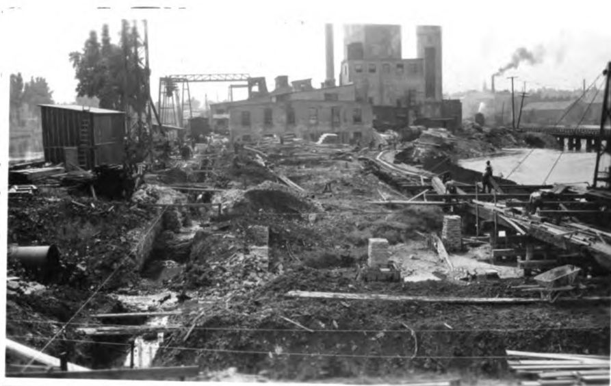
#3 July 30th, 1923. Excavating for south wall footings. Removing old trestle Driving Sheet Piling with steam hammer at extreme right.
