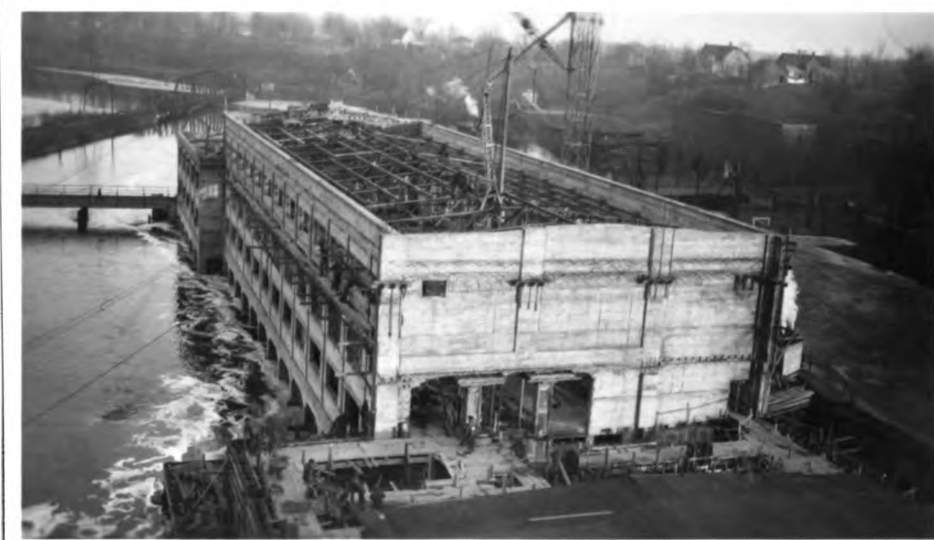
#28 Dec.18,1923. Forming stock building floor,(main) Setting roof steel in machine building.
