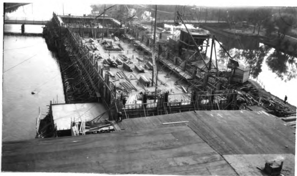
#20 October 8, 1923. Preparing to pour walls of finishing building in background. Note platform for concrete 'buggies'.
