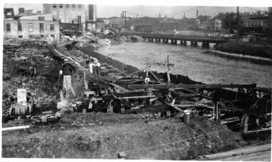
#4 August 2, 1923. Cofferdam completed and pumped out. Excavating for wall between machine and finishing bldgs.
