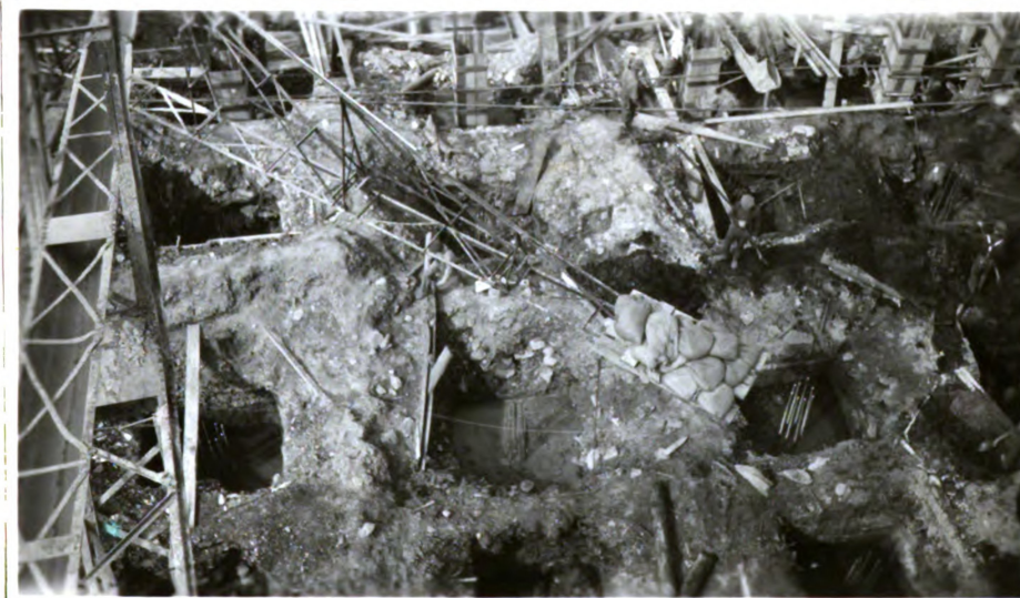
#12 August 23, 1923. View from tower of the footings of machine bldg. Re- inforcing dowels set in footings.
