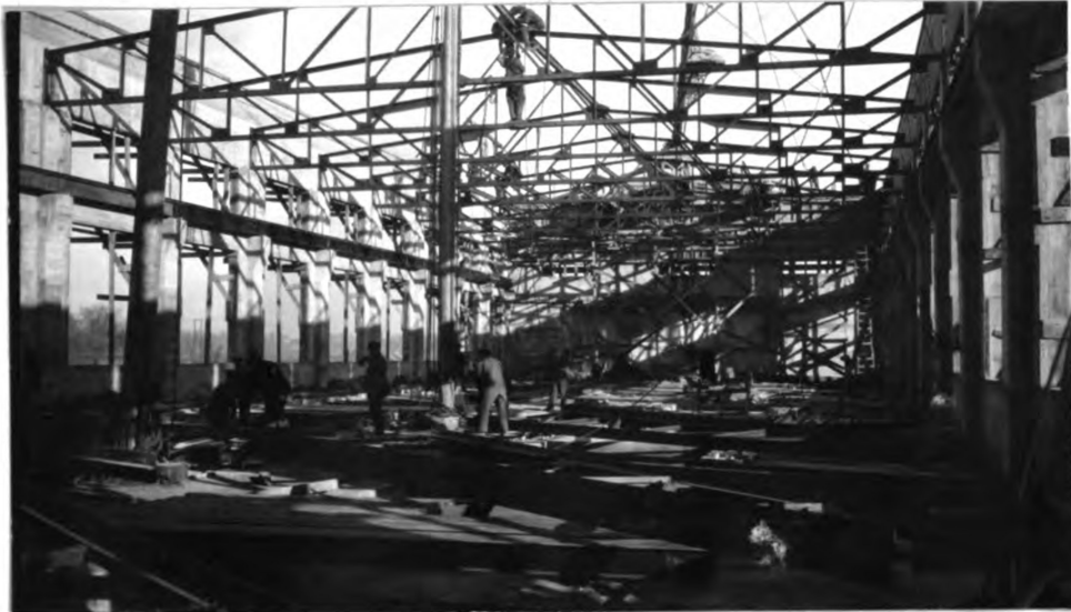
#27 Dec.15,1928. Bolting, riveting setting roof steel in machine building.
