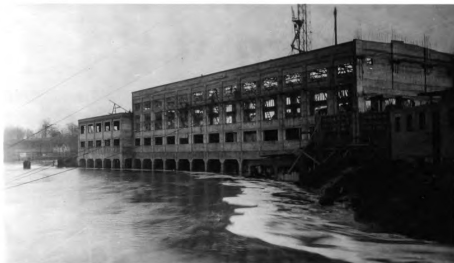
#30 Stock building walls being formed. View from the northwest. Setting steel sash.
