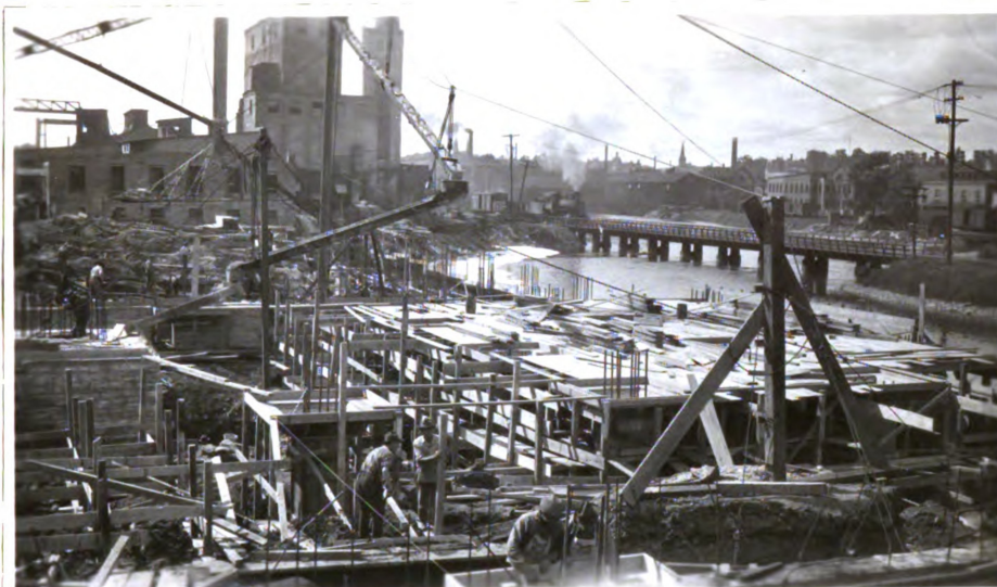
#11. August 23, 1923. Forming basement floor of finishing building. Note pier heads.
