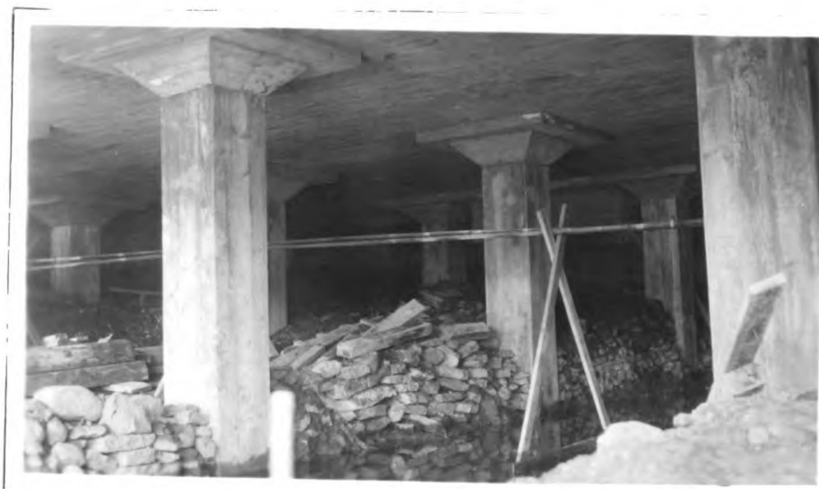
#19 Sept. 30, 1923. Piers under finishing building. Tailrace of water wheel in foreground.
