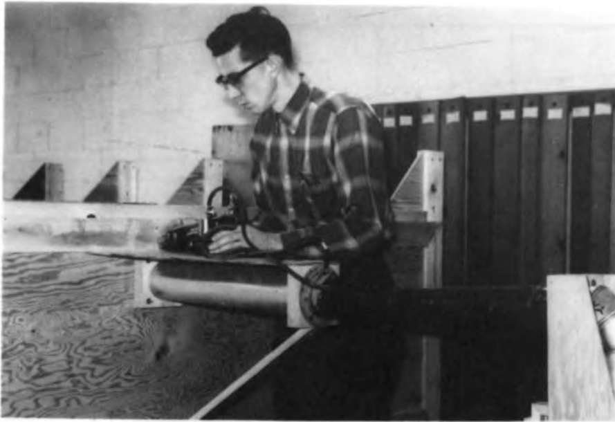
Figure 4.5. -- View at outlet end of chamber showing venturi and manometer.
