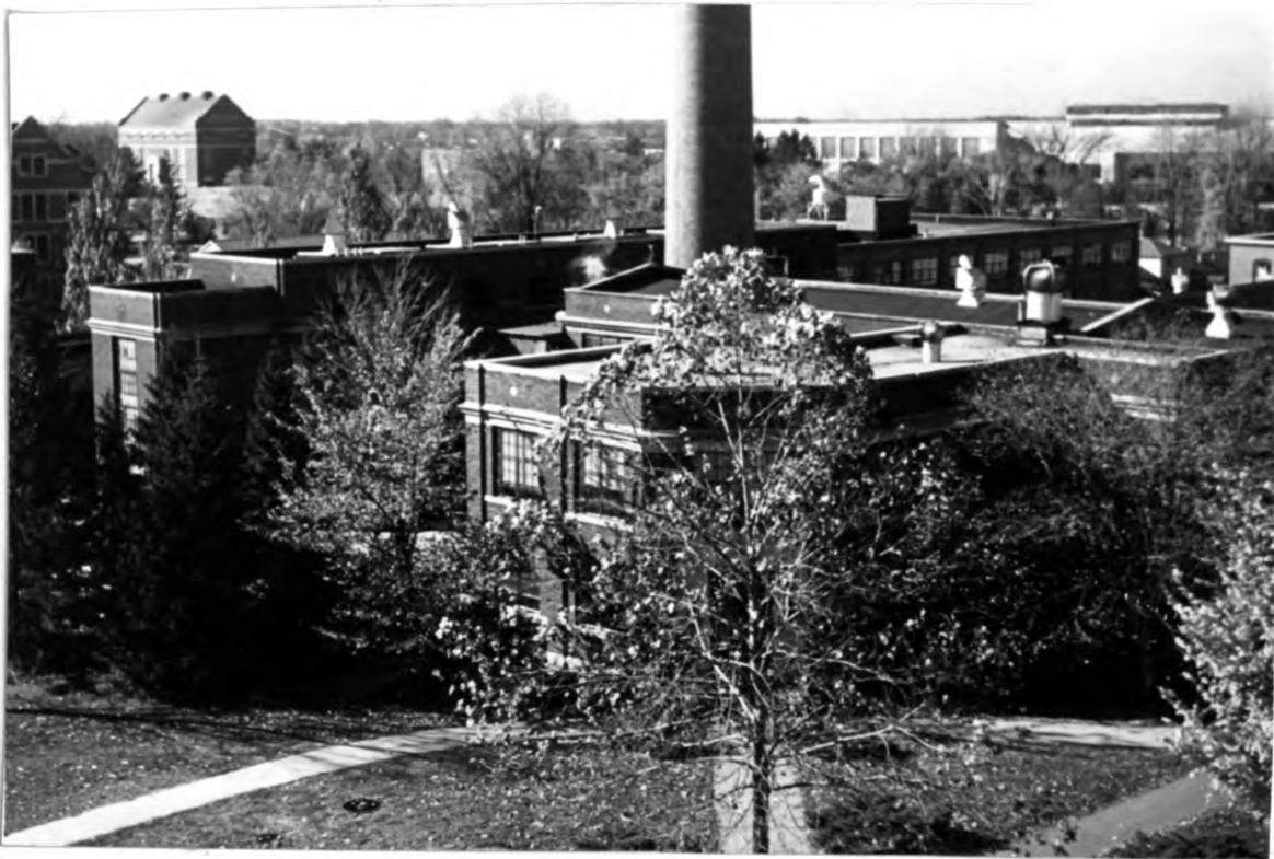
North Campus Power Plant. Note the South Campus Power Plant in the background.
